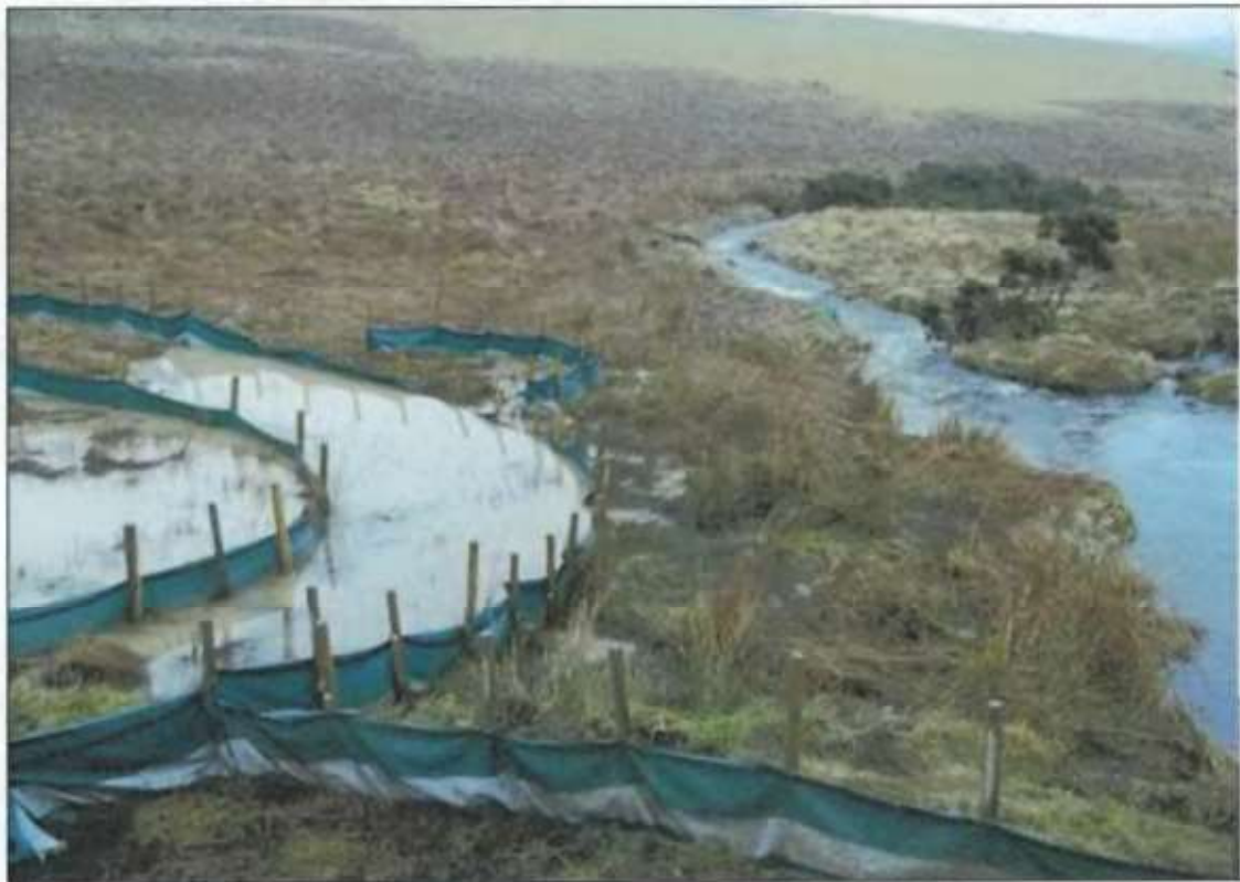
Plate 5.2: Photograph of silt fencing
