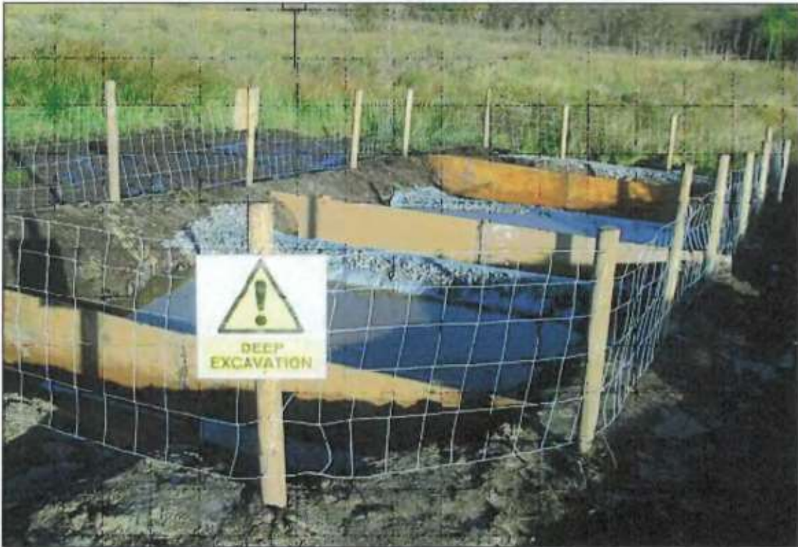
Plate 5.4a: Completed settlement pond system
