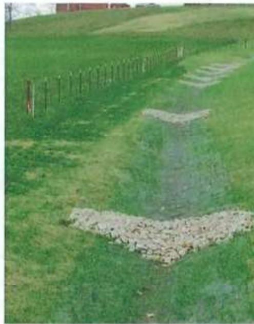
Plate 5.3: Photograph of Check Dams
